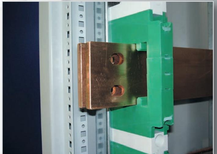
Busbars at 120 x 12 mm (160 x 10 mm on request) can easily be bent using a universal working cylinder, and holes of Ø 6.6 up to 21.5 mm including longitudinal holes can be punched through the simple insertion of hole punches
